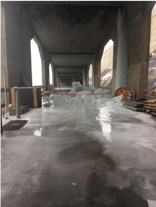
Photo 4: Access under the Ladder
